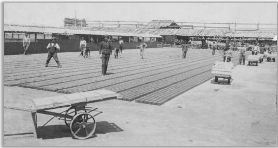
Drying bricks at the Thomas brickyard at Montague City. c. 1920s.
