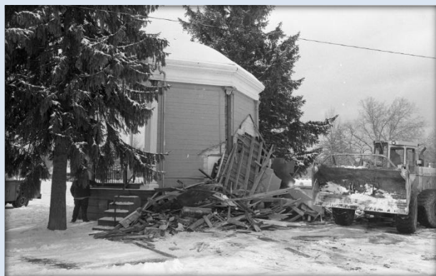
Unity Park Bandstand razing. e.g. archive
