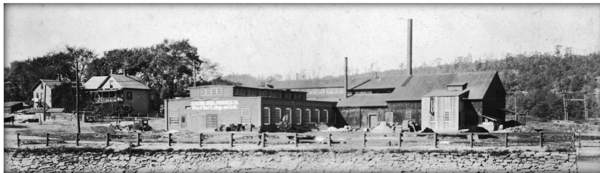
Electric Steel Mfg. Co. 1919. The former Hinckley Mfg. Co.
