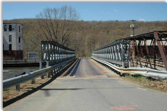
Bailey truss bridge. 3.26.06
