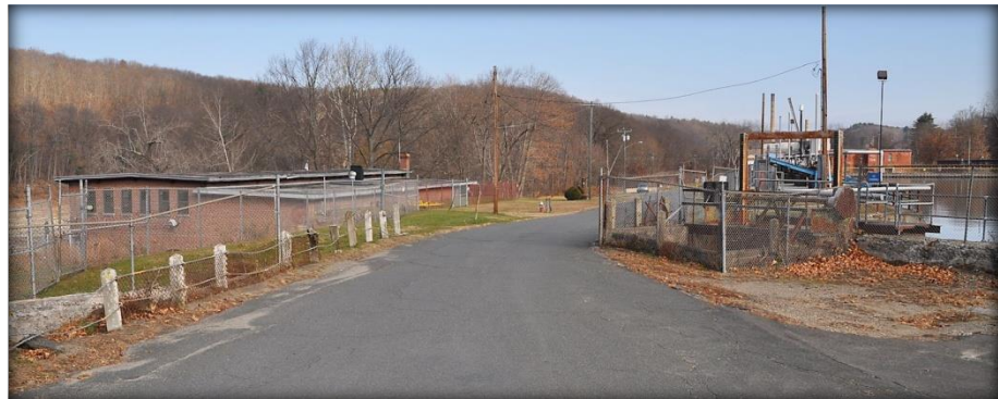
The location of the #1 "I" St. bridge. Looking north. 11.18.12
