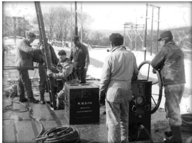
Joe Naida prepares to dive into the canal to inspect the gates that keep rubble from entering the penstocks at the No.1 Power Station at the Patch. 1956. Courtesy Mrs. Joseph Naida
