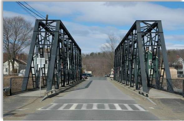
Eleventh Street Bridge-east portal. 3.26.06
