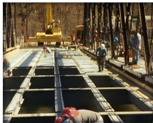
11th St. Bridge new deck, 1995. Courtesy Mitzi Croteau
