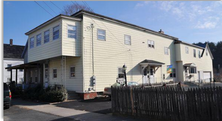
The rear of the Demers residence was a bakery. 11.18.12
