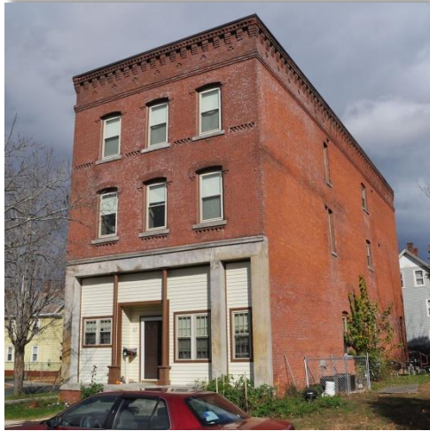
The Shanahan Block - home of the Hanover Club. Today the Franklin Community Action Group Neighborhood Youth Corps. is located on the ground floor. 10.31.10
