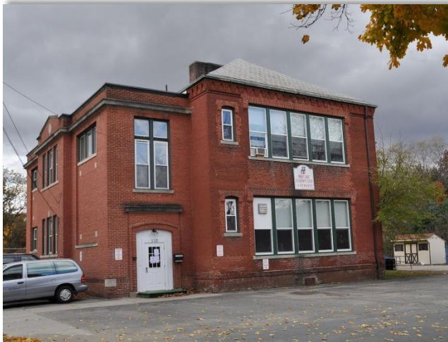
The north facade of the Patch School. Currently, the Parent-Child Development facility has offices here.
